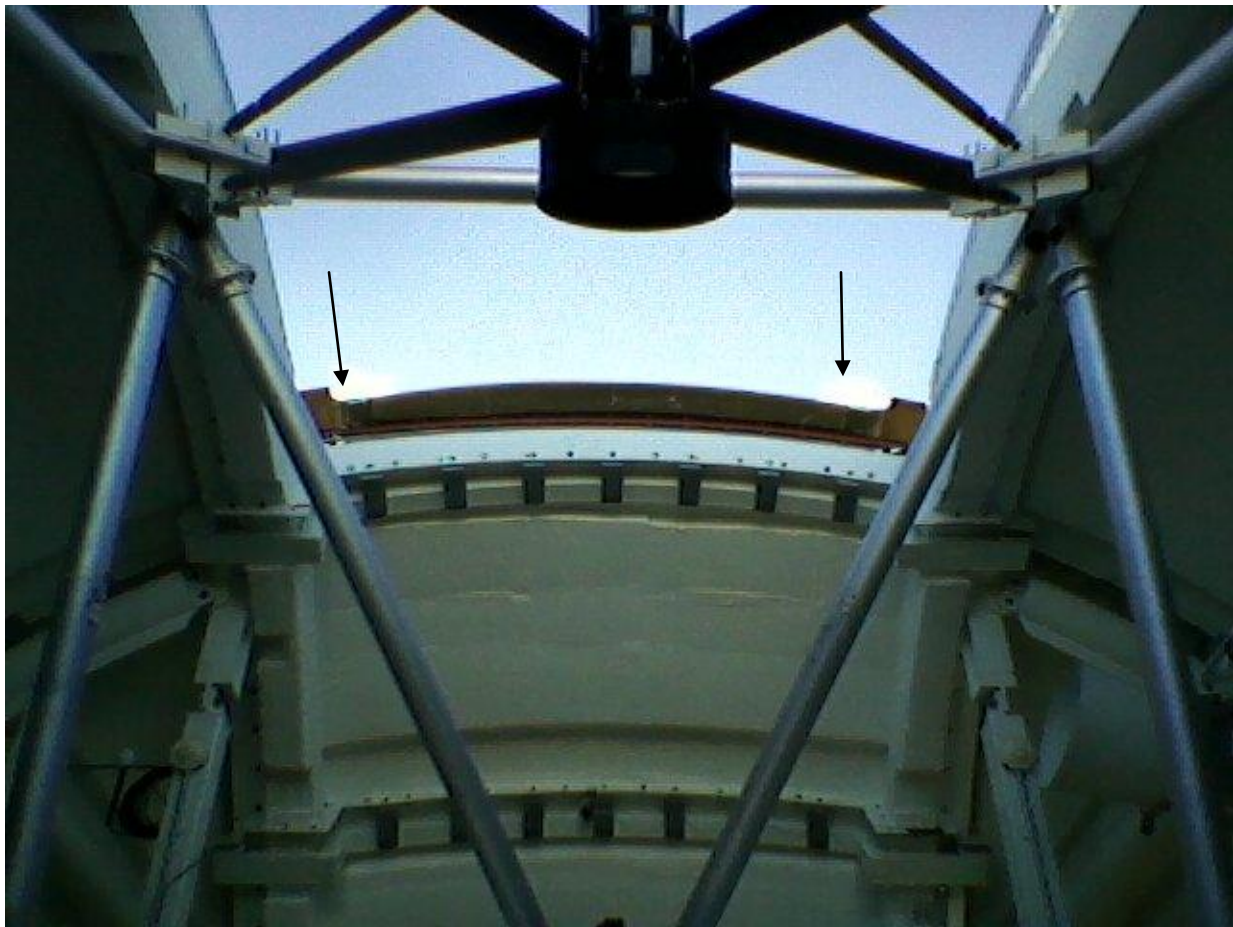
Figure 2.12: Shutter in open position showing chunks of ice.
