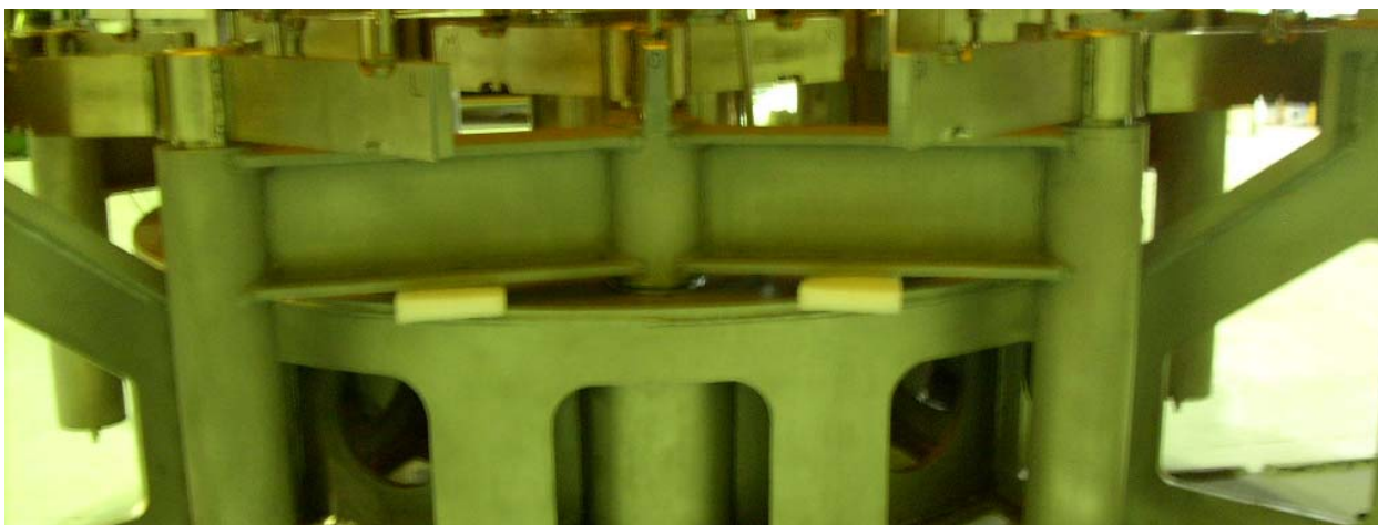
Figure 4-6 Foam Blocks installed under Main Loadspreader Assembly
