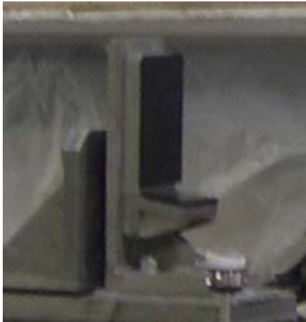
Figure 5-3 Seismic Restraint with SR Bracket 3 removed
