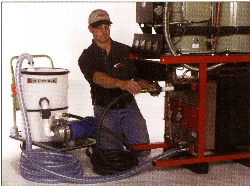
Figure 3: Inserting FlushGun into heat exchanger.
