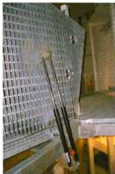
Second Strut re-installed
