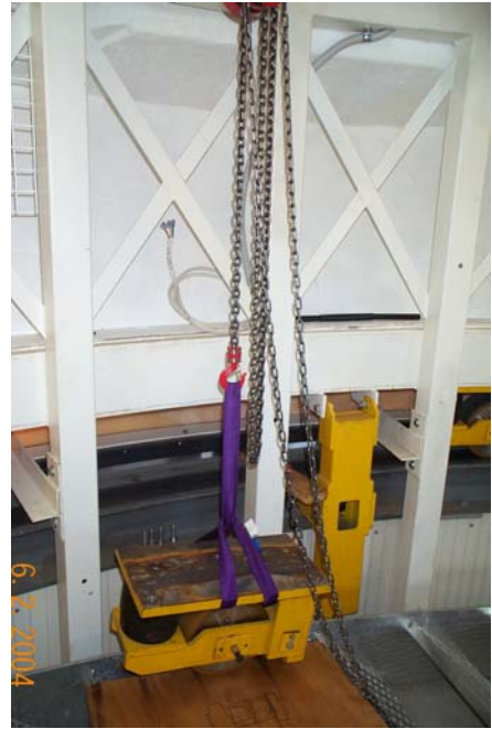
Replacing Bogey: Block and Tackle-Sling Arrangement
