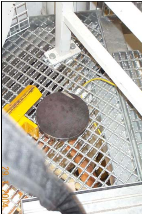
Azimuth Bogey Hard Point in Level 3 Floor
