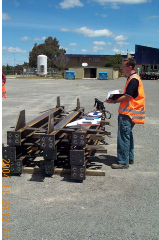
Figure 1-8 Ring beam columns
