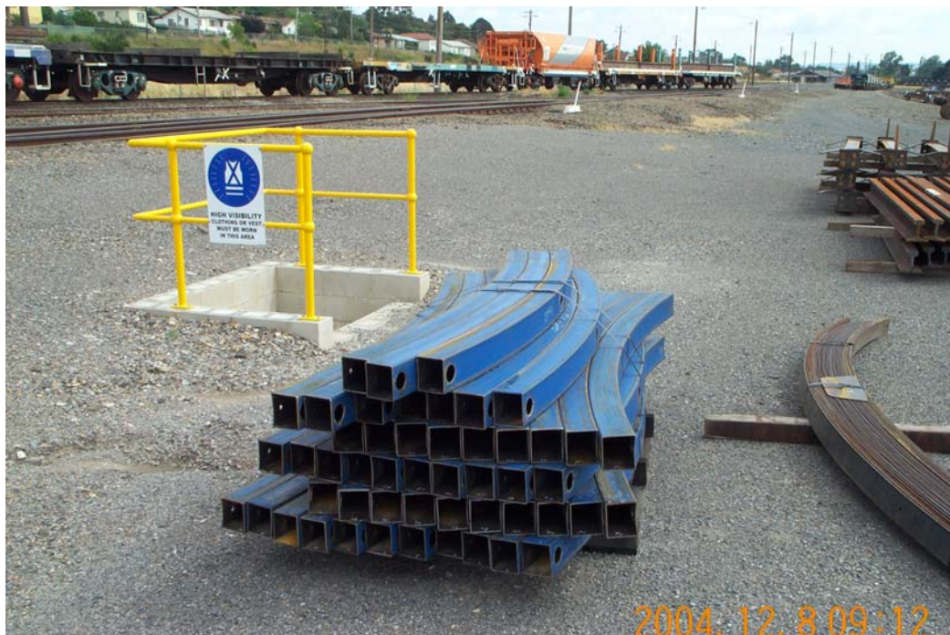
Figure 2-2 Horizontal outer girts
