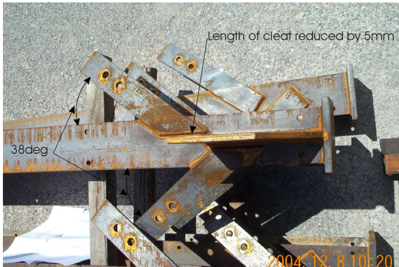
Figure 2-4 Balcony support columns
