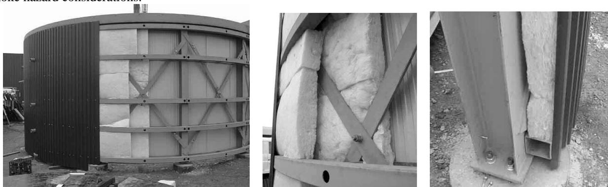
**Figure 10. Ring Wall Insulation Detail**
