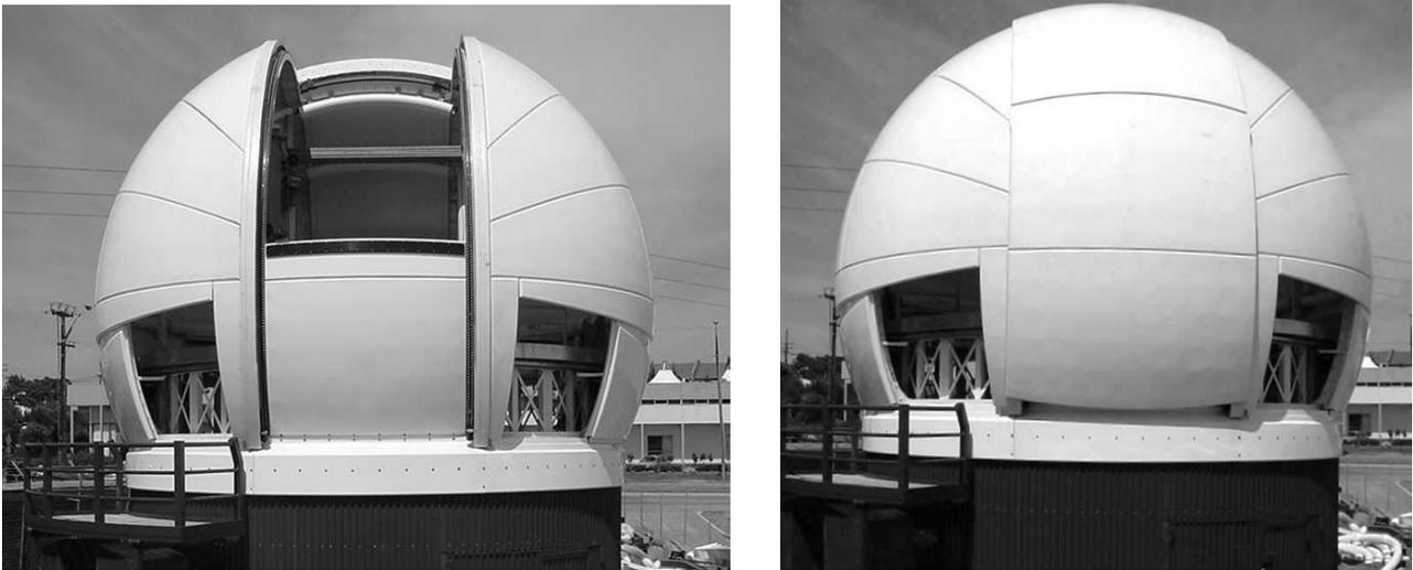
**Figure 11. IceStorm Series I Vent Doors Open Front and Rear**
